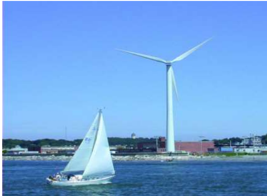
Figure : Typical Wind Turbine.
